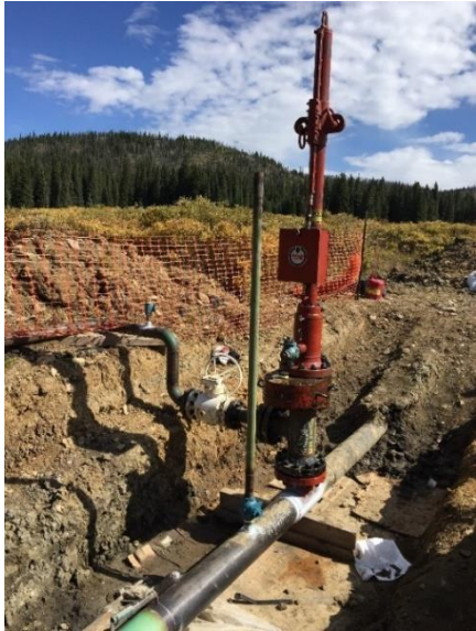
Stopper fitting and installation machinery, Courtesy of Xcel Energy.
