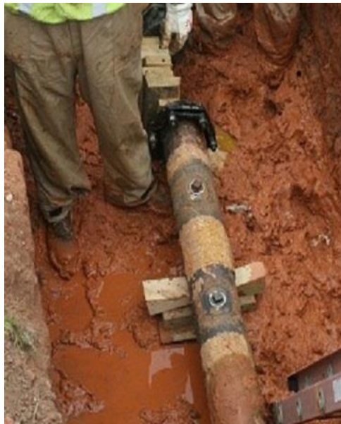
Photo of bagging completed, leaving two plugs, courtesy of David Payne, PLCS, LLC.
